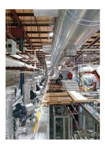
A recent project for Dijko Ovens saw a custom built concentric system specifically for the oven types designed by Dijko. Approximately 6% of the heat is recovered and used to supply heat back into the ovens, making the system exceptionally efficient.
