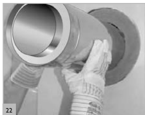
Example of a design with a double-walled connecting flue pipe.
